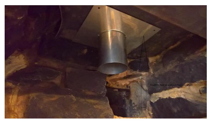
Stone fire place with brick chimney lined with 6" (150mm) flex. liner finished with a register plate adaptor. The gloss flue pipe slips over the outside of this. When finished it please email the height for the plate to the floor, so we can work out what flue pipe to bring.
